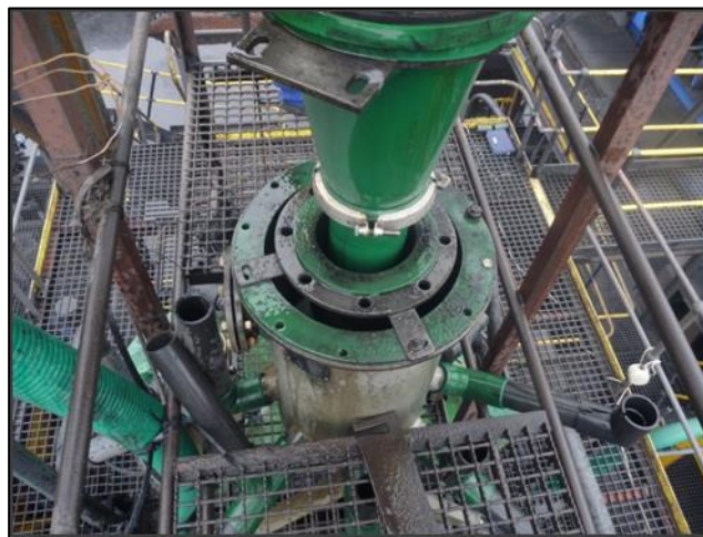
Figure 7: Desliming cyclone and spiral feed distributor installation
